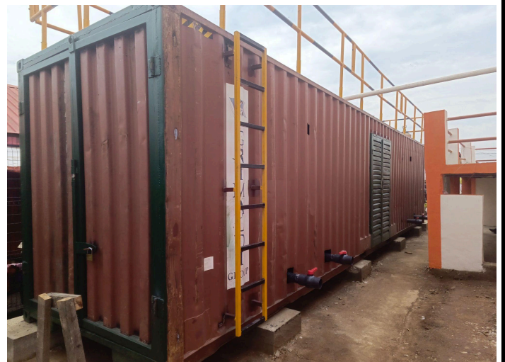
Figure 1: Biodigester installed at Ikosi fruit market in Lagos
