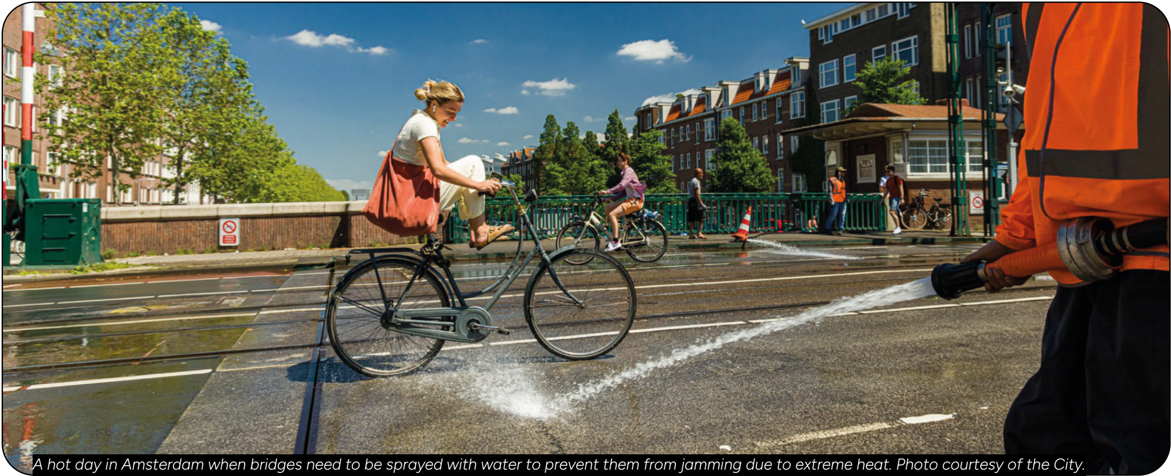
A hot day in Amsterdam when bridges need to be sprayed with water to prevent them from jamming due to extreme heat. Photo courtesy of the City.
